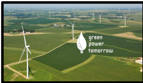
Farm field with wind and solar power
